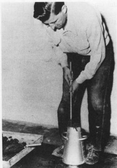
Rodding and filling cone using three separate layers of concrete
