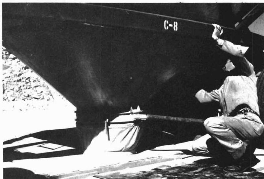
Figure 90.—Connection used in dumping cement from transport trucks to receiving hoppers of cement storage silos at Glen Canyon Dam, in Arizona. This arrangement minimized cement loss. P557-420-04599.
