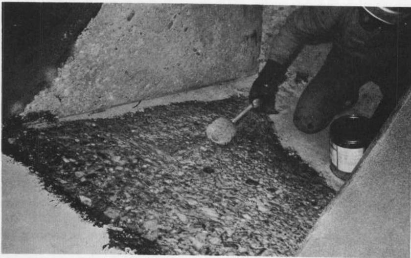
Figure 182.—Epoxy bond-coat being applied to sandblasted area adjacent to the dentates in Yellowtail Afterbay Dam sluiceway. Following this, epoxy mortar is placed over fluid or tacky epoxy to form epoxy-bonded epoxy mortar. P459-D-68900.
