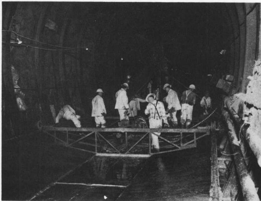
**Figure 142.**—Placing concrete with slip form in invert section of Spring Creek Tunnel No. 1, Central Valley project, California. P416-229-9608.
