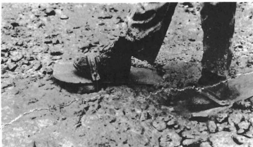
Figure 120.—Workman wearing “snowshoes” on a fresh joint surface. Snowshoes minimize undesirable working of the concrete and facilitate cleaning of the surface. PX-D-33053.
