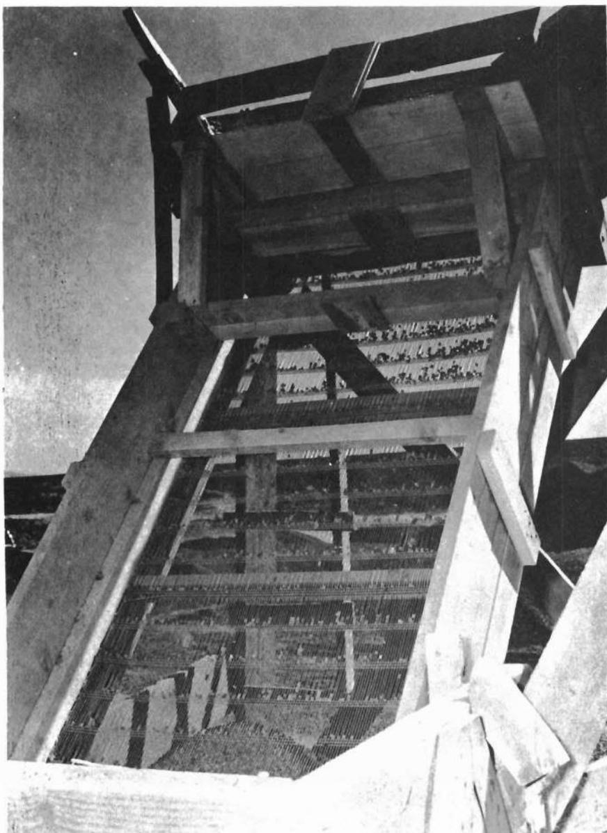
**Figure 87.**—Stationary screen with 3/16-inch by 4-inch slotted openings for finish screening coarse aggregate used on the Columbia Basin project, Washington. Note pile of undersize material visible through screen. CB-3702-4.
