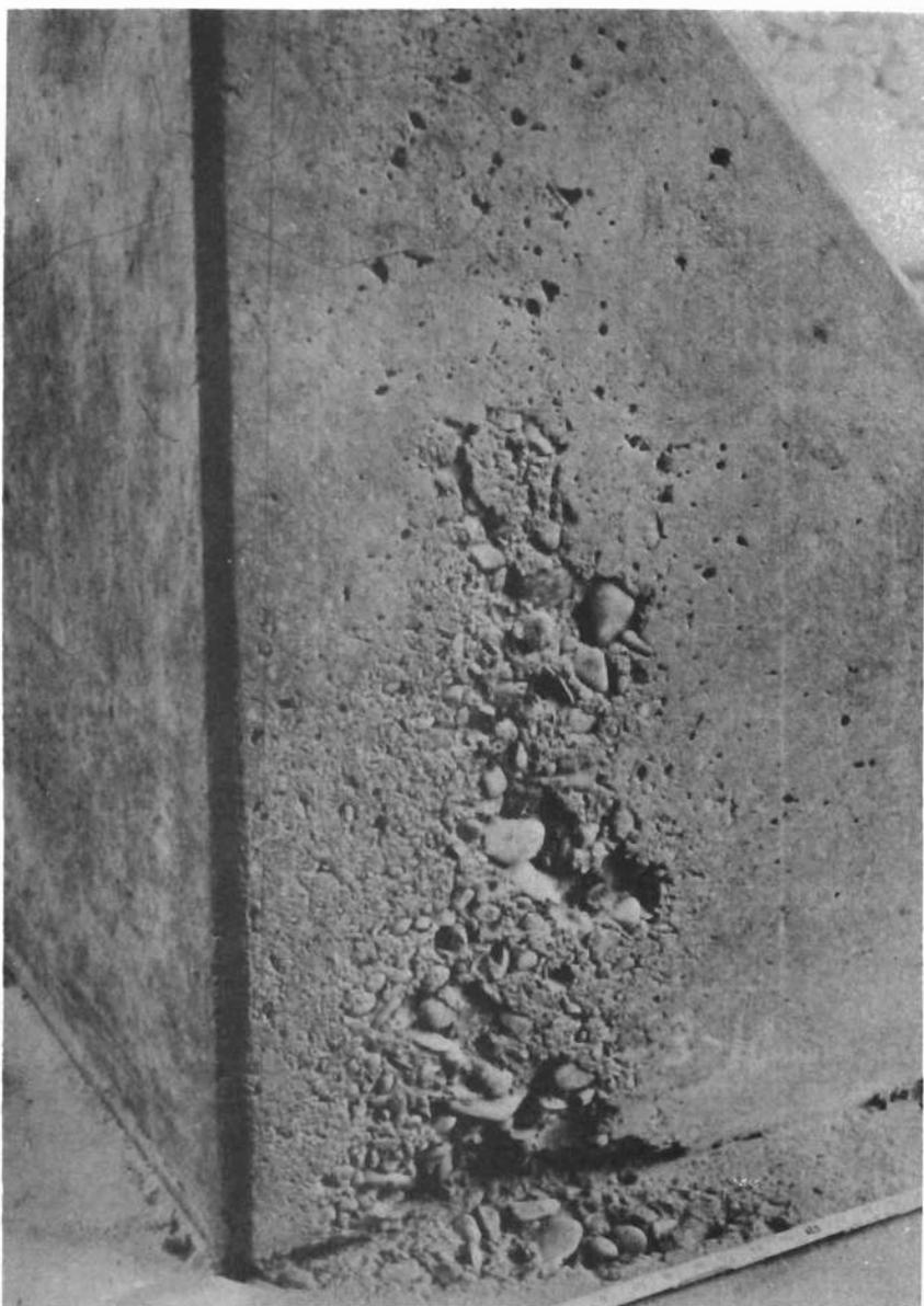
Figure 6.—Cavitation erosion of concrete on and adjacent to a dentate in the Yellowtail Afterbay Dam spillway stilling basin. Fast-moving water during a flood flow caused a pressure phenomenon at the concrete surface which triggered the cavitation damage shown here. P459-D-68902.
