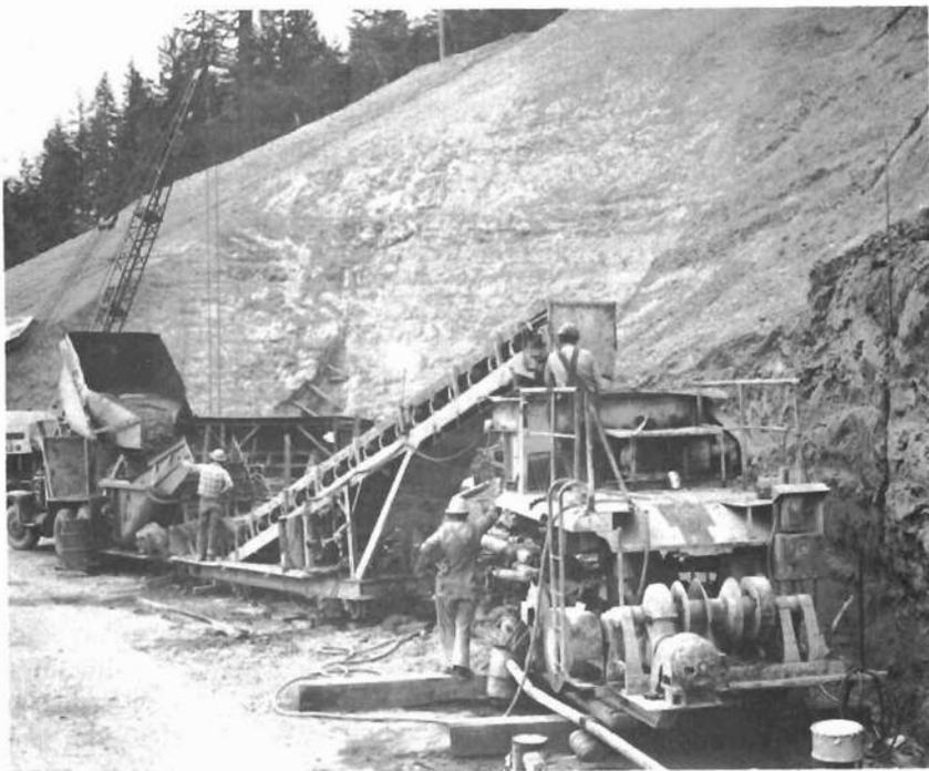
Figure 134.—Equipment and method used for pumping concrete into spillway tunnel at Trinity Dam, Central Valley project, California. TD-5008-CV.
