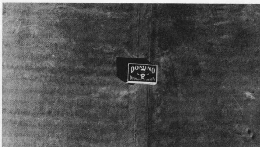
**Figure 199.**—Surfaces of concrete formed on an 0.8 to 1 slope at Shasta Dam, Central Valley project, California. Upper and lower pictures show surfaces produced by wood forms and vacuum forms, respectively. PX-D-33060.
