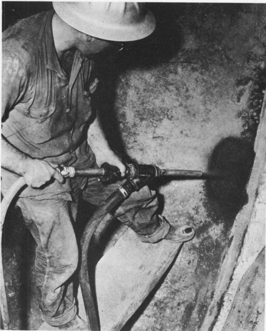
**Figure 181.**—Application of replacement mortar. The mortar should be applied on dry contact surfaces that are as clean as a freshly broken piece of concrete. PX-D-33057.
