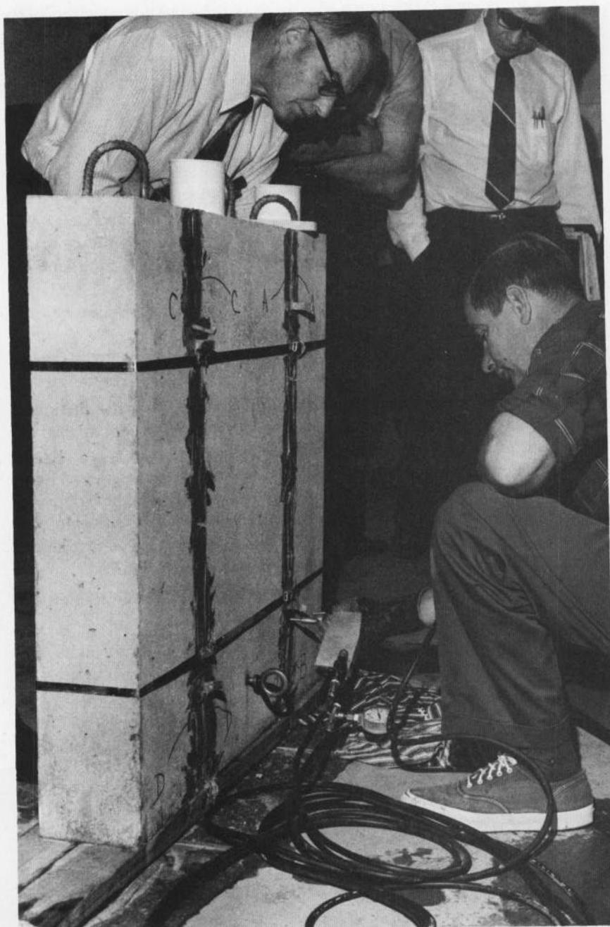
Figure 187.—Demonstration of a proprietary epoxy grout injection system for repairing cracks in concrete structures. P801-D-75011.
