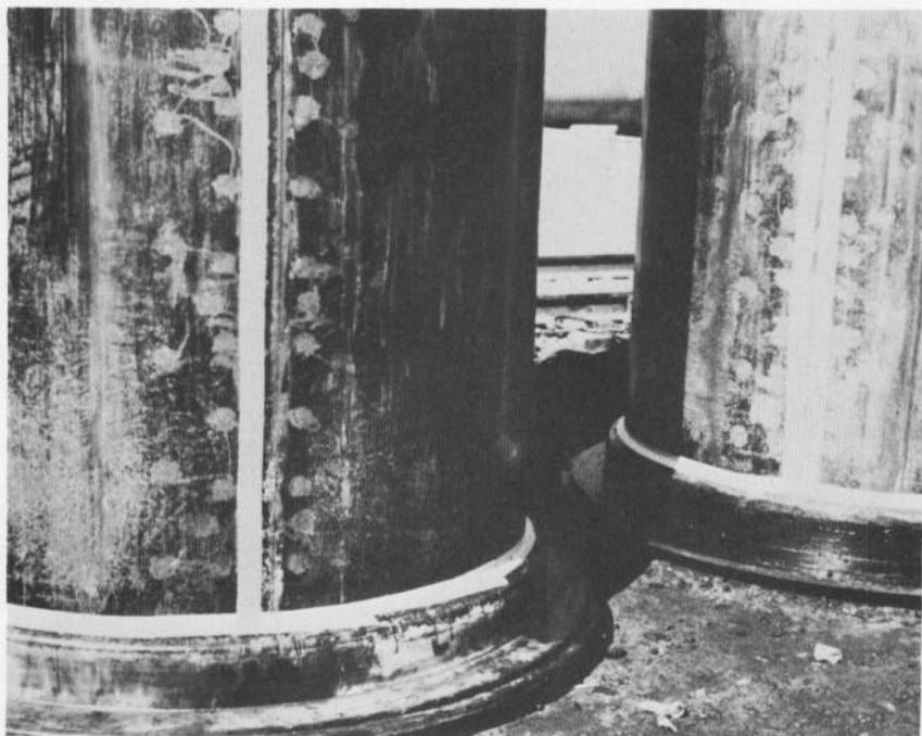
Figure 162.—Forms for cast pipe. If tight gaskets are not used in form joints, gates in inside forms and joints with base rings should be sealed with 2-inch cloth tape that will adhere firmly throughout the placing operation. Paper tape is not fully satisfactory. PX-D-34610.
