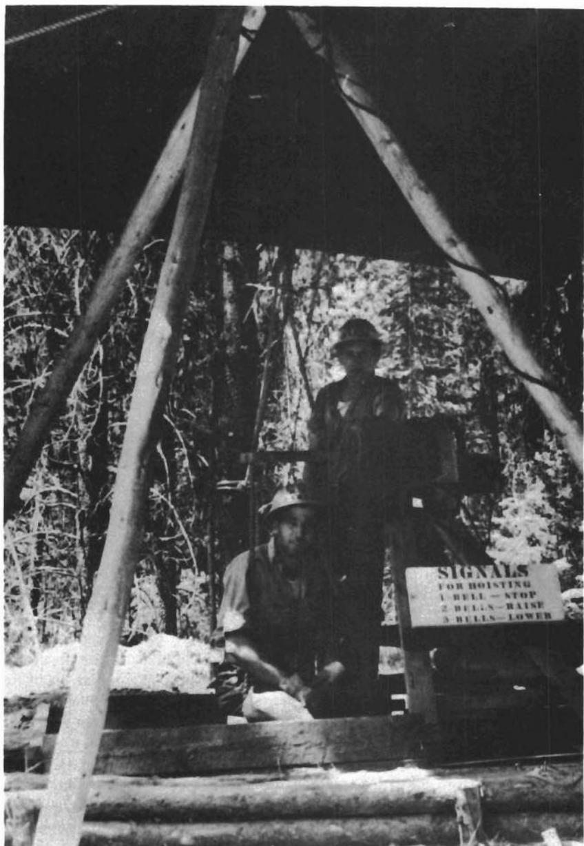
Figure 45.—View of test-pit collar setup. PX-D-32045.
