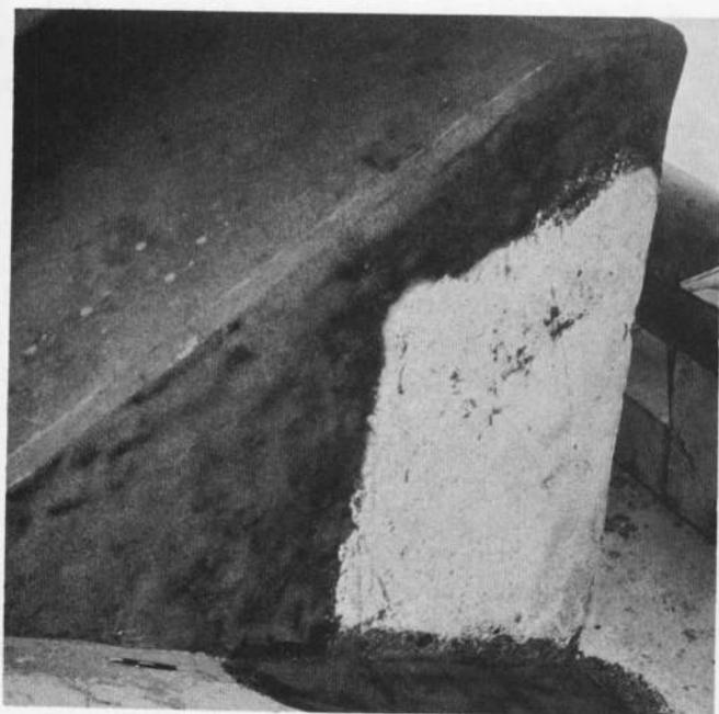
**Figure 184.**—Epoxy-bonded epoxy mortar repairs. In upper photograph epoxy mortar is placed on epoxy bond-coat previously applied to wall of sluceway at Yellowtail Afterbay Dam. The lower photograph shows a dentate in sluceway repaired with epoxy-bonded epoxy mortar. The difference in mortar color in the two photographs is caused by use of different colored sands. P459-D-68911 (upper), P459-D-68912 (lower).
