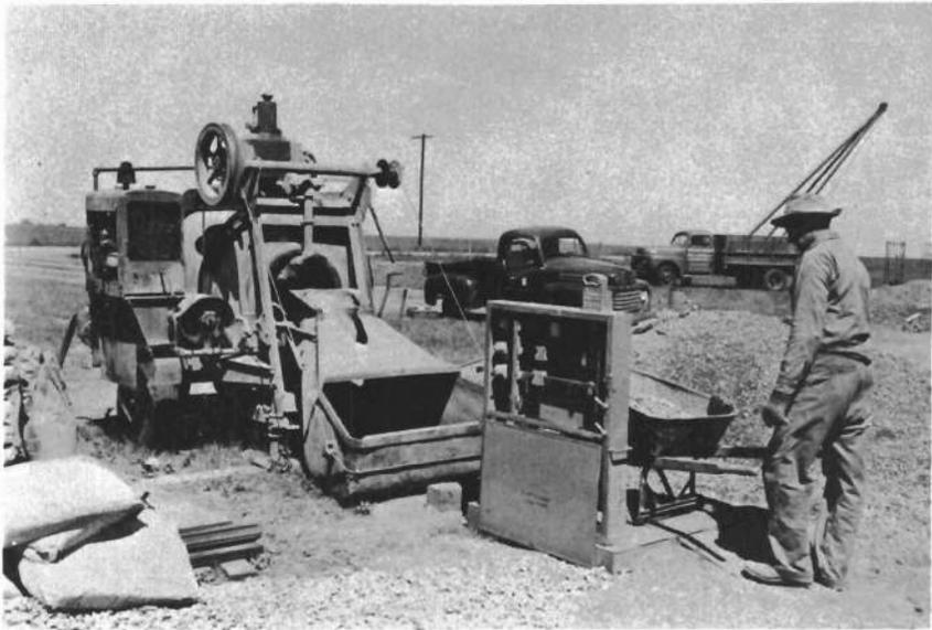
Figure 107.—Batching concrete by means of a portable wheelbarrow scale. Use of such equipment permits securing uniform concrete on the small job. 466-602-604.
