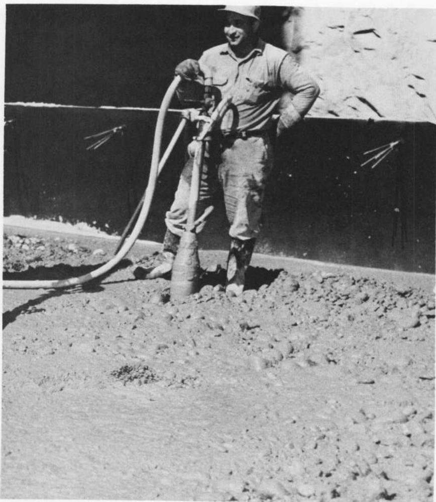
**Figure 140.—Concrete after proper consolidation. Note that workman stands on concrete despite its appearance of wetness. P557-420-08212.**
