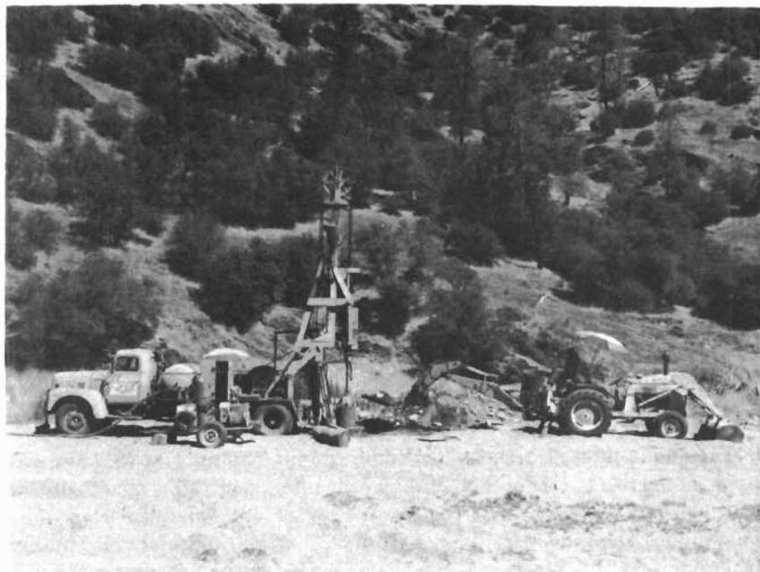
Figure 39.—Clamshell excavator and backhoe unit with reverse shovel exploring the gravel bars at Auburn Dam, California. P1859-245-5533.
