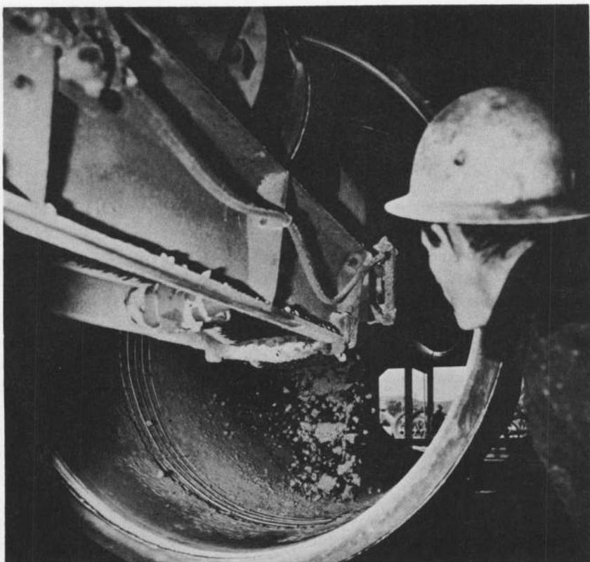
Figure 165.—A centrifugal method of manufacturing concrete pipe in which the concrete is also directly compacted by a steel roller. PX-D-34070.
