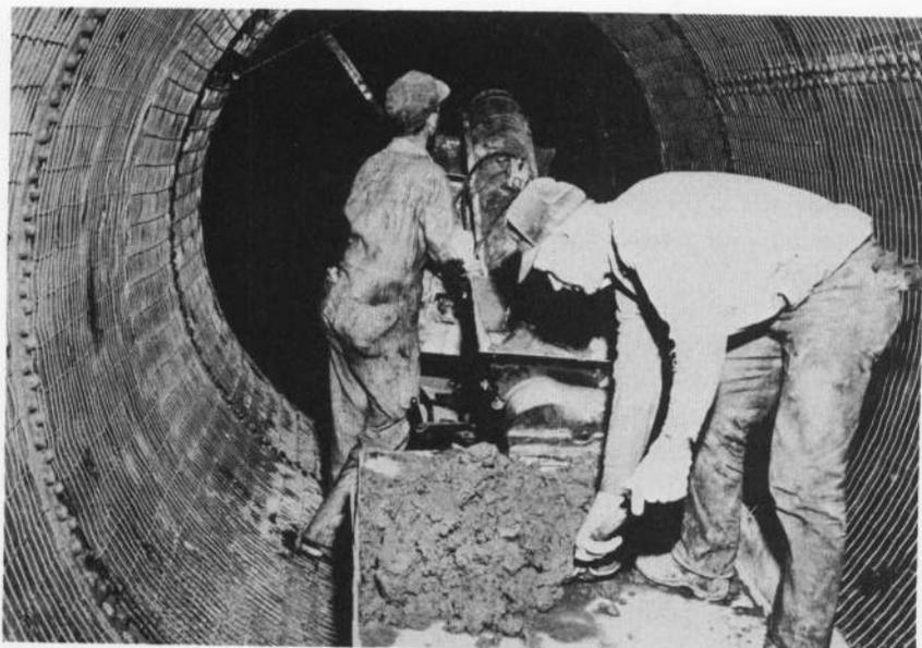
Figure 205.—Workmen shoveling mortar into a lining machine which will distribute it over the interior surface of a steel pipe. Reinforcement has been fastened to the surface to strengthen the lining. Normally, the lining is placed without reinforcement. P126-100-19.
