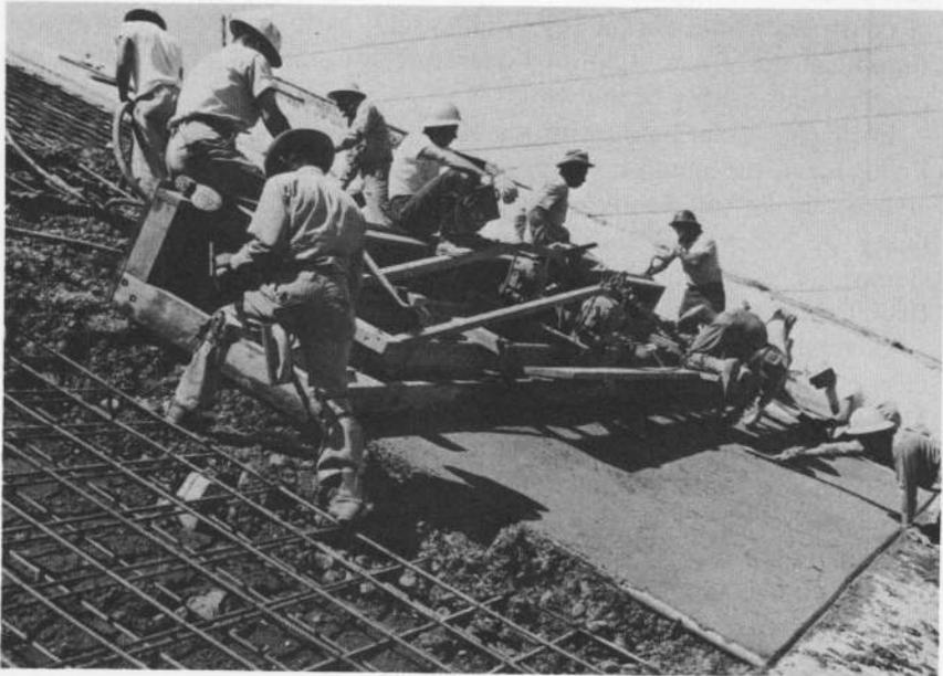
Figure 145.—Job-built slip form being used on sloping apron of left abutment of Nimbus Dam, Central Valley project, California. Reinforcement is systematically tied and supported on concrete blocks. Notice pattern formed by using V-grooves at construction joint of abutment in background. AR-1523-CV.
