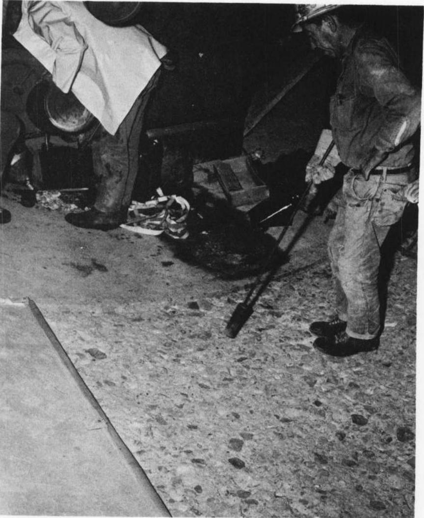
**Figure 177.—A gas-fired weed burner being used to warm and dry an area prior to the placing of epoxy-bonded concrete in the spillway tunnel at Blue Mesa Dam, Colorado River Storage project. P622A-427-15030.**
