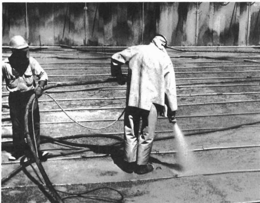
Figure 121.—Final sandblasting of construction joints at Glen Canyon Dam, in Arizona. This is an expeditious and effective means of construction joint cleanup. P557-420-05101.
