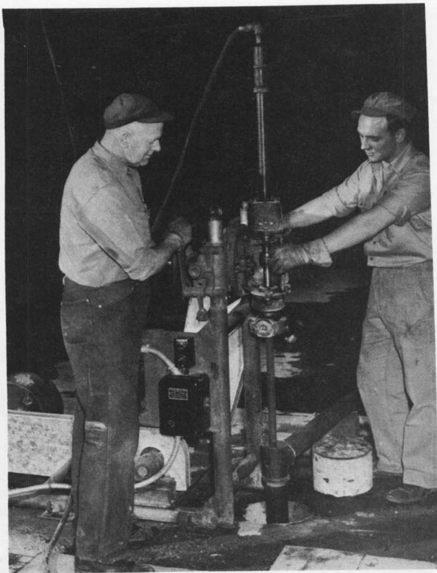
**Figure 207.—Drilling a 10-inch core in concrete floor. PX-D-33518.**
