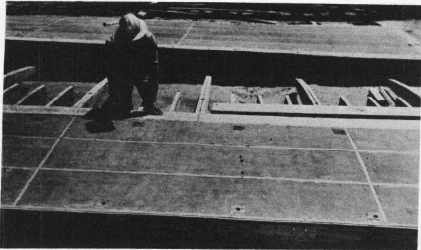
Figure 201.—Vacuum panels being constructed at Angostura Dam, in South Dakota. View shows rubber strips and hardware cloth before covering with muslin. PX-D-33514.
