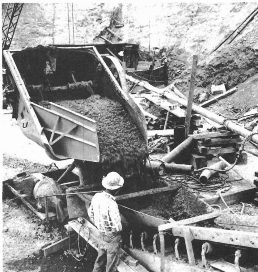
**Figure 114.—Dumpcrete bed being used to discharge concrete into feed hopper of a belt conveyor. Note agitator in bed which largely eliminates segregation of material. 214—TD—5010—CV.**
