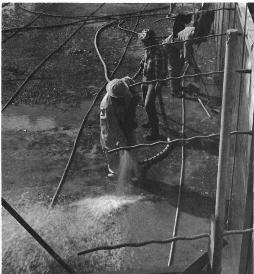
**Figure 122.—Final washing with water jets just prior to placing next lift of concrete. P1222-142-11967.**
